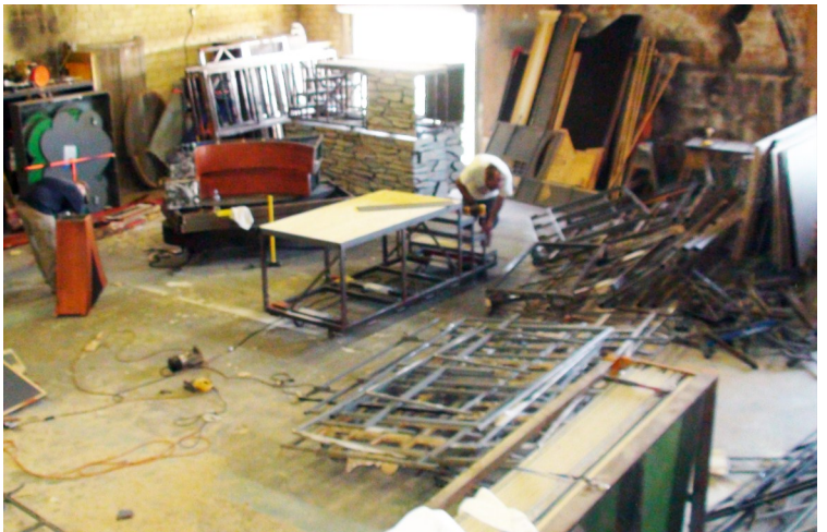
*Separating steel from wood for recycling
